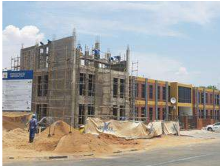
East wing construction in progress
